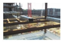
The Decking Contractor will usually ensure that the manufacture of the decking is coordinated in separate bundles for each bay of steelwork. Each decking bundle should be loaded out onto the bay where it is to be installed; this greatly reduces the risks associated with working at height and the amount of manual handling required.
